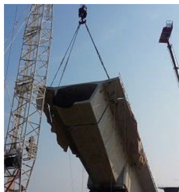
Taking Apart the Concrete Bridge
