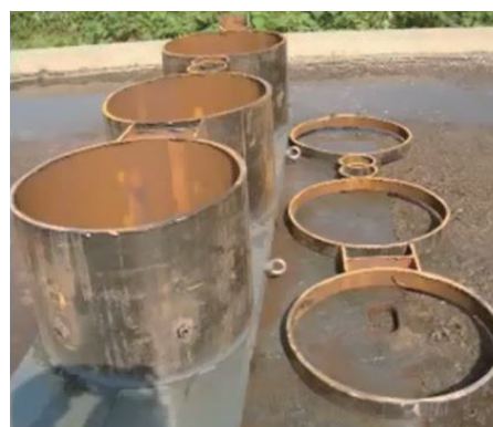
Steel Pipe Sheet Pile Cutting
