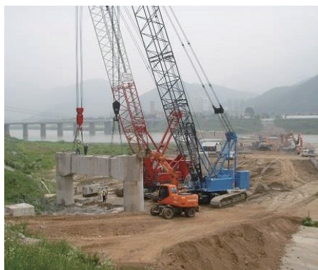
Disassembling the Concrete Bridge
